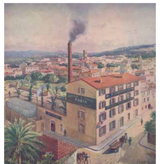
View of the former Robertet factory Engraving from a supplement to the Revue des marques de la Parfumerie et de la Savonnerie (Journal of Perfume and Soap Industry Brands) 1924, Grasse
