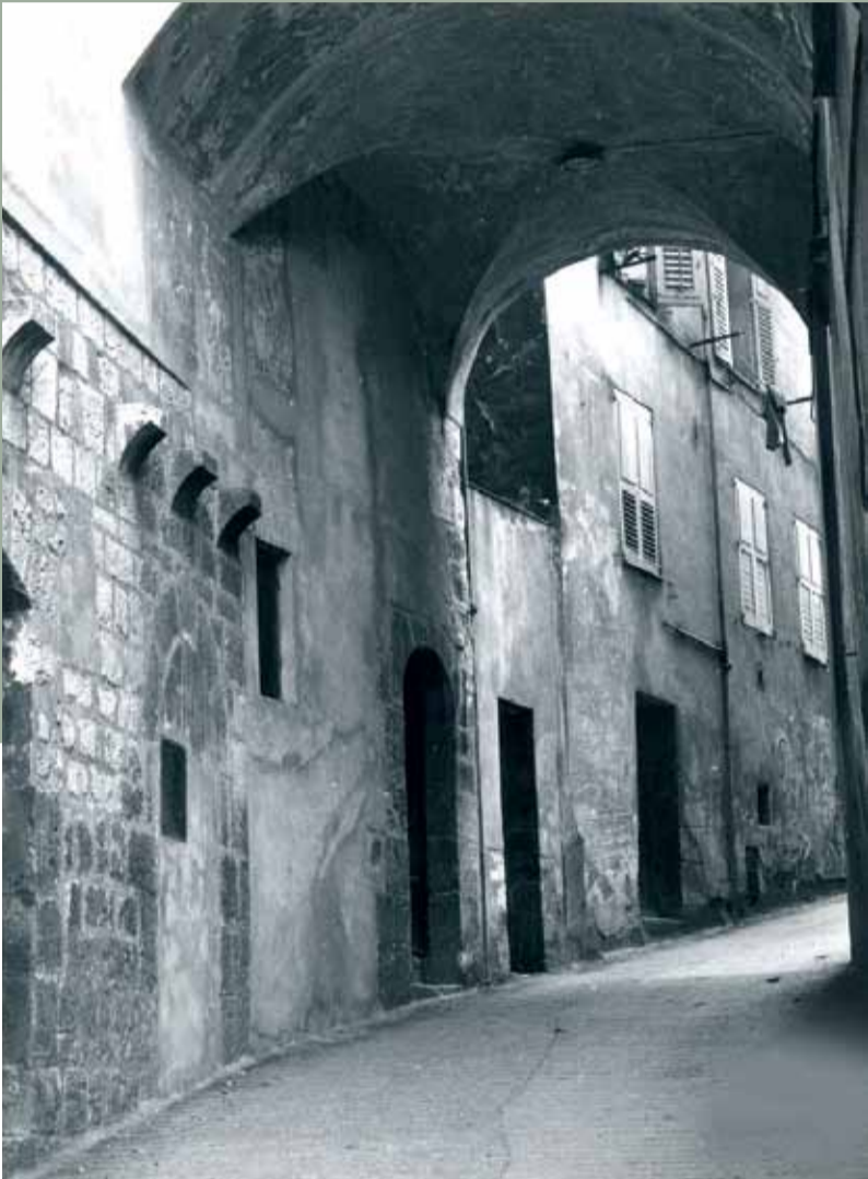
Medieval house 2007, Grasse, Rue Tracastel
